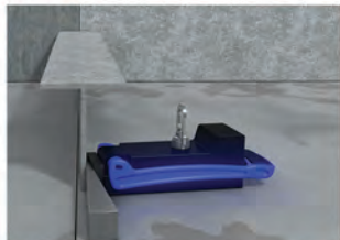
2. Place Magnet Wedge Block and wedge
